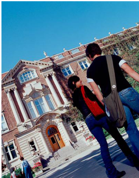
Arts Building, University of Alberta
